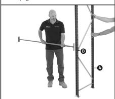
4 Add a second support beam <sup>(b)</sup> to the uprights <sup>(c)</sup> at the same height and ensure beams are knocked in fully with a rubber mallet
