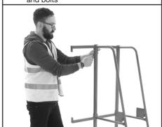
Attach the end upright A to the beams B by checking correct alignments and then securing with nuts and bolts. Once frame is complete, fully tighten all of the fixings.
